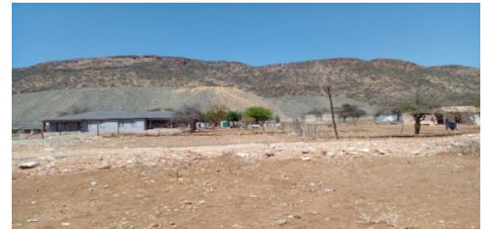
Blast vibrations causes damages in homes near Bauba Platinum Mine
